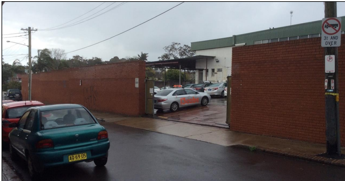
Image 3: The Site as viewed from Union Street
